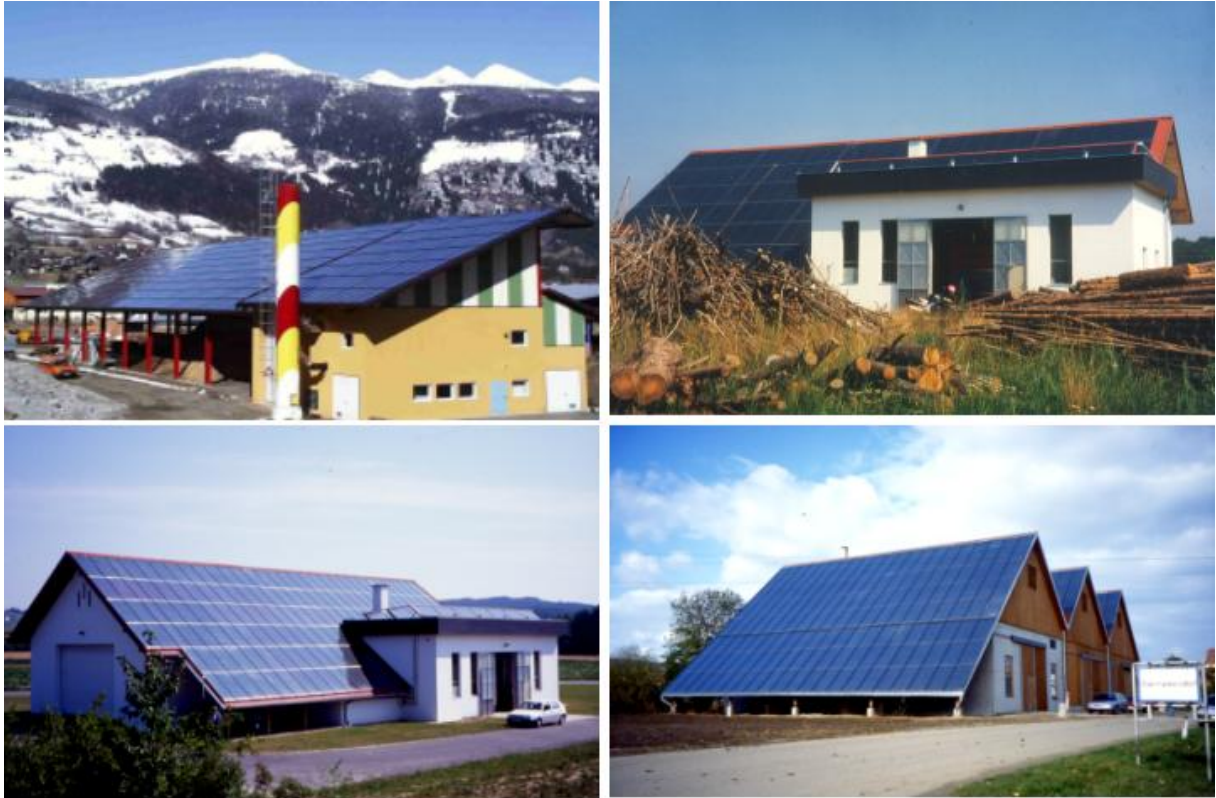
Fig. 14a: Solar-combined biomass district heating: Projects in Austria
