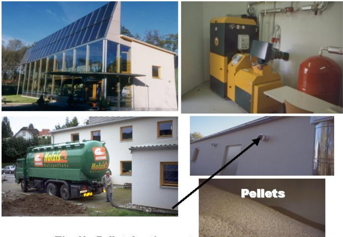
Fig. 9b: Pellets heating system for housing estates
