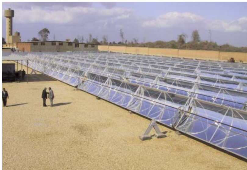
Fig. 7: El NASR Pharmaceutical Chemicals, Egypt. Installed capacity: 1,33 MW th Source: Fichtner Solar GmbH. Germany.
