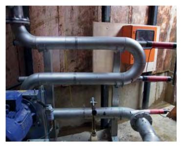
**Figure 13:** Electrokinetic disintegration unit (photo and unit by Atres, Germany)
