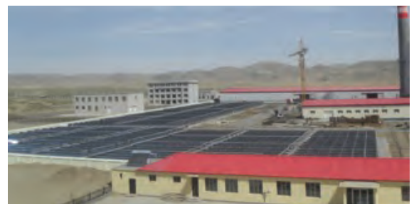
▲ Top to bottom: Solar combisystem in a Beijing suburb. Solar cooling system in Hainan Province. Solar industry process heat at a print & dye factory in Jiangsu Province. Solar district heating system in Inner Mongolia autonomous region.
