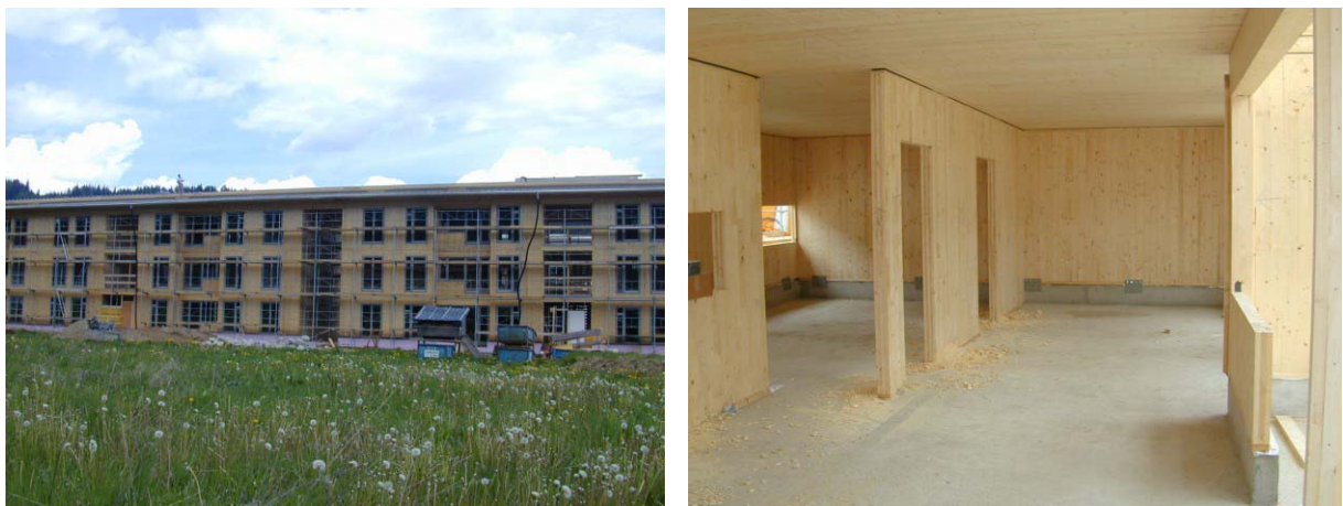
Fig. 1: Residential building, Judenburg West, Austria; wood as main construction material (Source: JOANNEUM RESEARCH)
