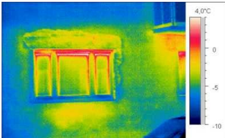
Fig. 6: Thermal imaging picture of a building construction in need of thermal refurbishment
