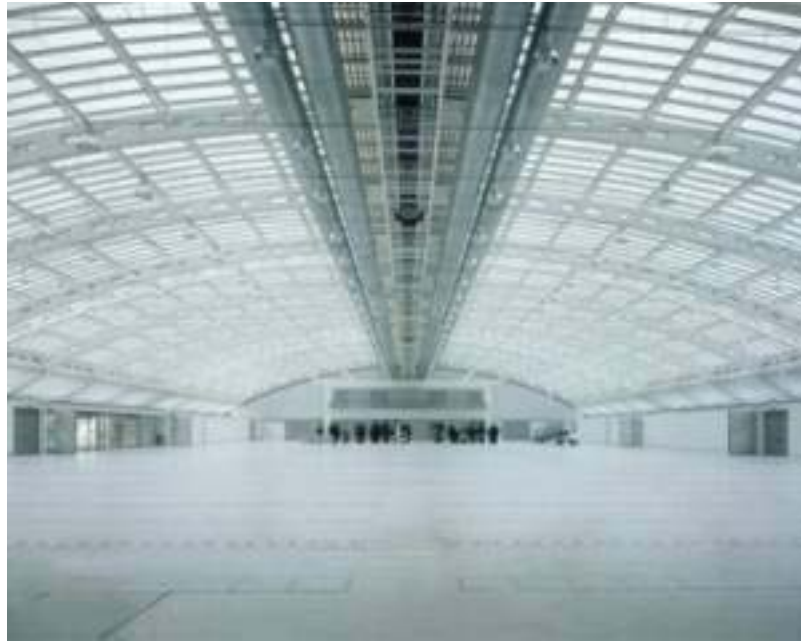
Fig. 5: Optimised use of natural daylight with the help of sun protection screens in the “Design-Center” in Linz (Foto: Bartenbach)
