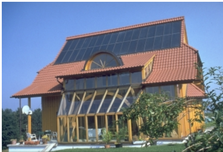
Figure 17a: Single family house with solar space heating
