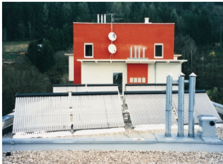
Figure 7: Vacuum-tube collector
