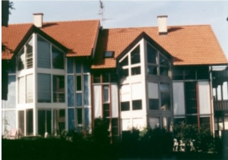
Figure 21: Terrace house estate with TWD - facade
