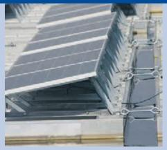
Fig. 1 - Floating PV Power Plant (INFINI Hyogo Daikyu Power Plant) (Inami Town, Hyogo Prefecture). Multicrystalline silicon PV module: 250 W x 6 846 modules (by INFINI) 1,7 MW.
