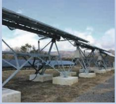
Fig. 3 - Fukushima Airport Mega-Solar Power Plant (Sukagawa City, Fukushima Prefecture, etc.). Total: 1,2 MW (500 kW, 200 kW, 500 kW), 30 types of PV modules including tracking system and various types of mounting structures.
