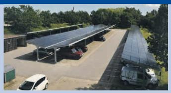
Fig. 1 - Car park with a 152 kWp PV system from the town hall in Fredensborg. Developed by Solar Park.
