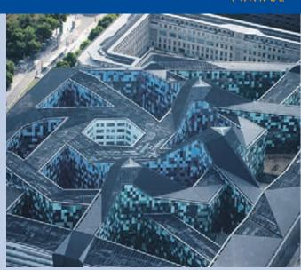
Fig. 2 – 820 kW BIPV rooftop with specially designed zinc coloured c-Si PV modules similar to zinc roofs in Paris (Photo: ANMA, ©R. Nicolas-Nelson/Armée de l'Air).
