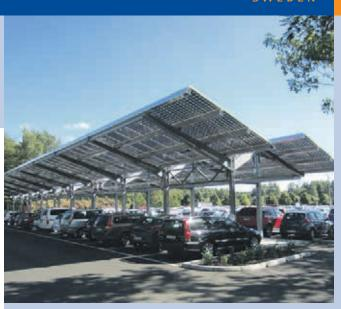
Fig. 3 - First stage on a planned 700 kW PV installation on roofs over a car parking, at Skaraborg Hospital (Photo: Johan Paradis).
