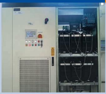
Fig. 3 - Li-lon Energy storage system (16 kWh) for 14 kWp grid connected PV plant on Lampedusa island (Photo: ENEA, <u>www.enea.it</u>).
