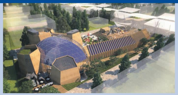
Fig. 1 - The roof of the Belgian pavilion at the Universal Exhibition in Milano was covered with BIPV laminated photovoltaic glass from the AGC Company (either crystalline photovoltaic cells or an organic fill).
