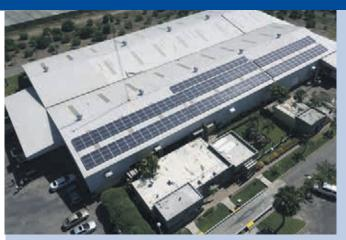
Fig. 1 - 70 kW PV System in a Fruit Packing Plant, Colima MX (Photo: Conermex).
