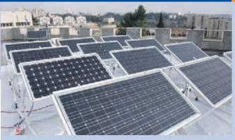
Fig. 1 - First generation BiFacial PV system installed by SolAround, with white background to increase the contribution of the back side of the PV panel. Overall efficiency of SolAround BiFacial panels is expected to be between 25-28 %.
