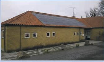
Fig. 4 - Roof integrated PV system by Storløkke holiday centre in Bornholm. A part of the PV Island Bornholm R&D project. Developed by Nielsen El, Rønne.
