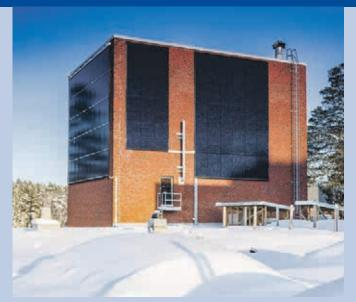
Fig. 1 - Wall-mounted solar PV panels at LUT (Photo: Lappeenranta University of Technology <u>www.lut.fi</u>).
