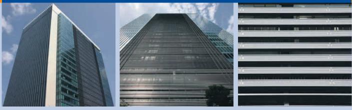
Fig. 2 - Office building "Ochanomizu Sola City" (Chiyoda Ward, Tokyo). Single crystalline silicon PV module: 150 kW.
