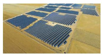
Fig.1 - The largest PV system in Turkey with the installed capacity of 18,5 MW (expected 30,7 GWh annual electricity generation) in Konya (still pending approval for grid connection) [10].
