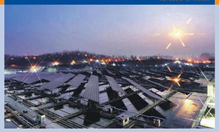
Fig. 3 - 5 MW PV power plant at Amsa Arisu Water Filtration Center, Seoul, Korea (Photo: Hankook-Ilbo).
