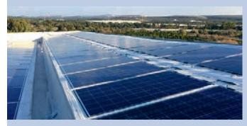
Fig. 2 - Solatics PV Integrated Membrane installation, using the "Direct Attachment" method.
