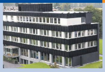
Fig. 5 - PV rooftop and façade systems on an office building in Flums (Photo: © NET Ltd. / DanielForster.com).
