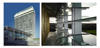
Figure 1: External View of the refurbished building (left) and detail of retrofitted second skin with automated glazed louvres (right)
