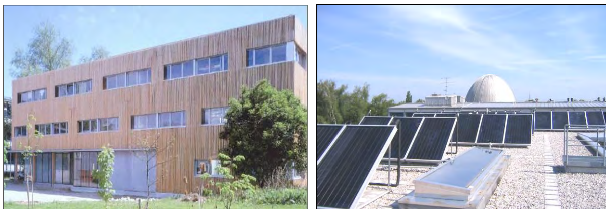
Figure 3: ZAE Bayern office building and solar thermal flat plate collectors on the rooftop
