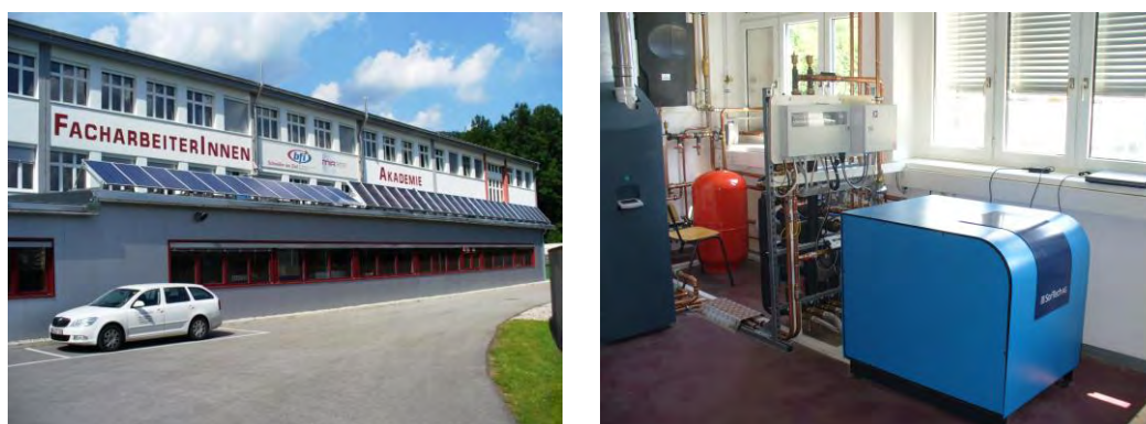
Figure 3: Solar Cooling Professional School, Mürzzuschlag, Austria (left: Solar thermal collector; right: Adsorption Chiller ACS08)
