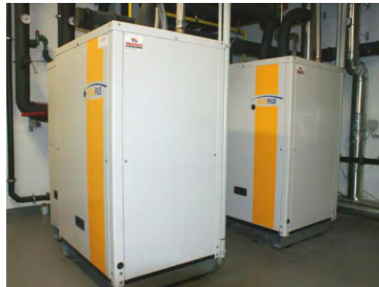
Figure 2: Photo of AHP installation
