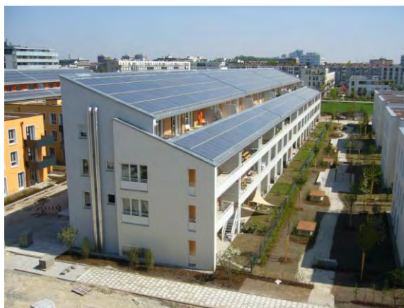
Figure 1: Picture of a building at Ackermannbogen showing a part of the solar system
