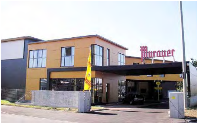
Figure 1: Storehouse building where the AHPs are installed
