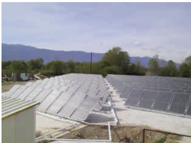
706 kW solar thermal plant for a dairy in Greece
