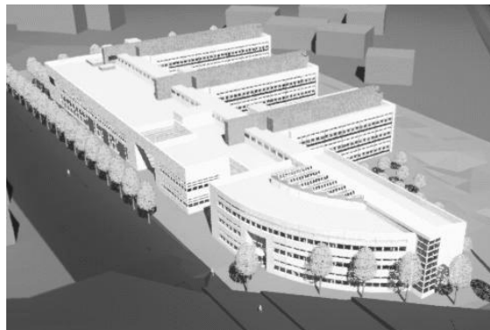
Fig. 2: Visualisation of the detailed design on the basis of the 3-dimensional CAD model and lighting simulation with RADIANCE, south-western aspect.
