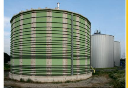
environmental advantages: 90 % less CO<sub>2</sub> is released during production. The resulting concrete is more resistant to acid and resists chemical attack much better than the material previously employed. It is no longer necessary to apply a coating to the inside of the digester; here again, material and expense are saved.
