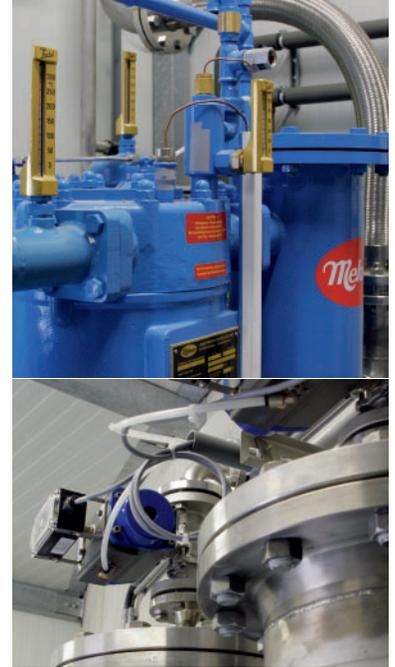
constituent is retained under pressure and passes to the high-pressure compressor at the filling station. The proportion of methane and carbon dioxide in the gas delivered („methaPUR“) is continuously analysed online, with feedback to the process. Provided that gas purity is up to standard, the biogenic methane stream is compressed to up to 300 bar for sale at the CNG pump. The biogas processing unit plus biogenic CNG filling station in Margarethen am Moos
