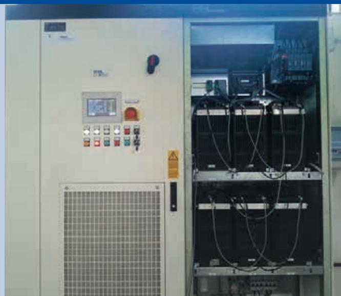
Fig. 3 - Li-Ion Energy storage system (16 kWh) for 14 kWp grid connected PV plant on Lampedusa island (Photo: ENEA, [www.enea.it](http://www.enea.it)).
