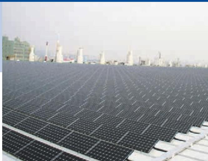
Fig. 2 - 3 MW roof mounted PV system at LG Electronics, Gumi-si, Gyunsangbuk-do, Korea (Photo: Solar Today).
