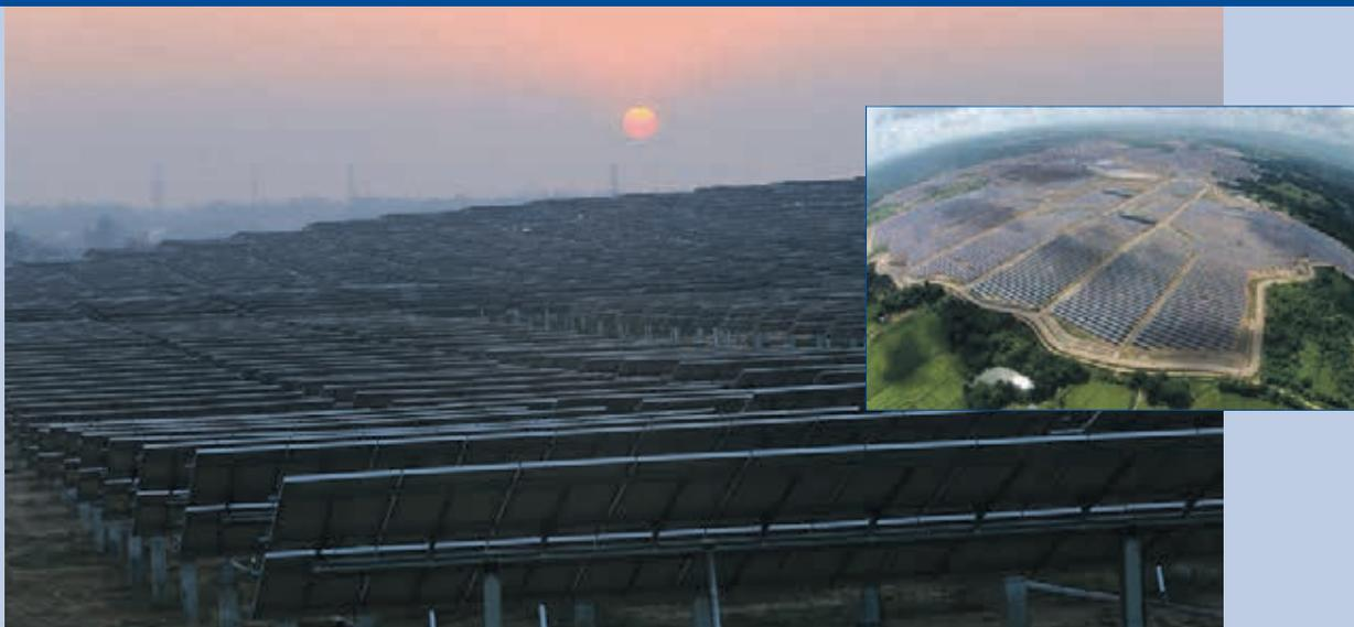
Fig. 3 - The Biggest SPP Project in 2015. This project has achieved COD since February 2015 in Lamphang province. Total installed capacity 126,396 MWp with Poly Crystalline Solar Cell, Solar Tracking System (Photos: Energy Absolute Public Company Limited).
