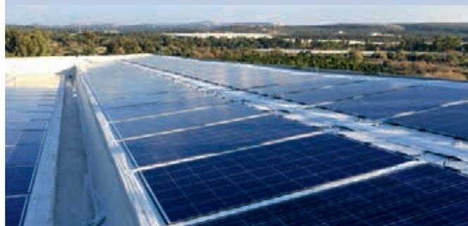
*Fig. 2 - Solatics PV Integrated Membrane installation, using the "Direct Attachment" method.*
