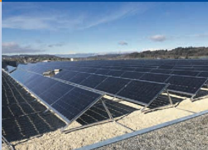
Fig. 2 - Self-consumption 658 kW PV system on a MIGROS supermarket with bifacial glass-glass modules, Schönbühl (Photo: Genossenschaft Migros Aare).
