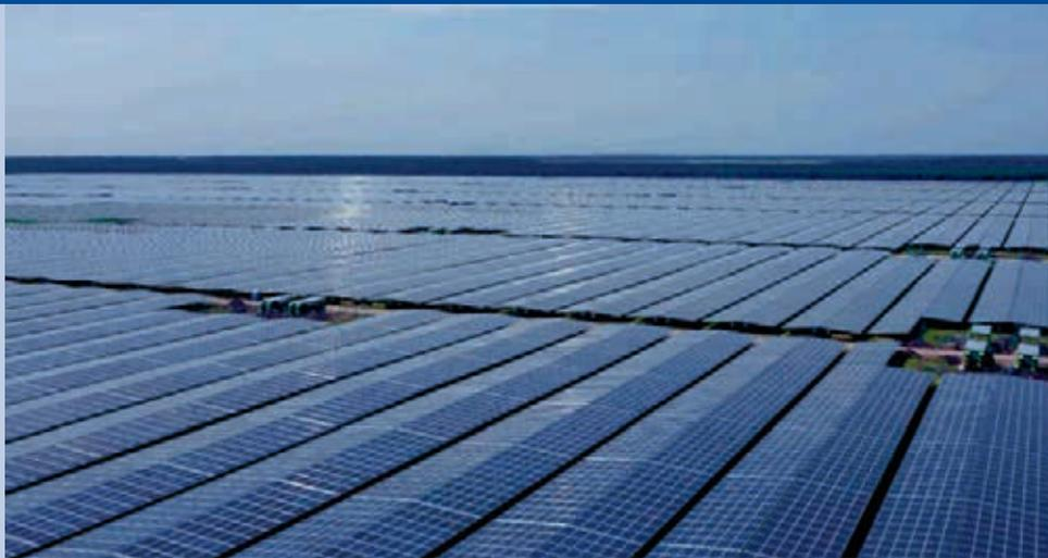
Fig. 3 – 230 MW PV plant, near Bordeaux, mounted on fixed structures with an east-west orientation (Photo: Neoen, Clemessy).
