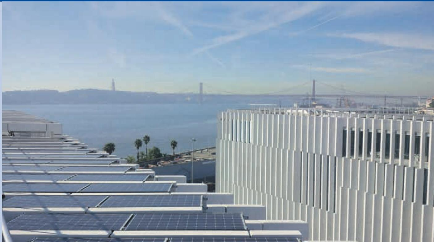
Fig. 1 – New EDP Headquarters in Lisbon – 84 kW PV self-consumption.
