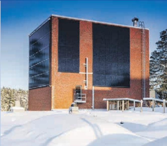
Fig. 1 - Wall-mounted solar PV panels at LUT (Photo: Lappeenranta University of Technology [www.lut.fi](http://www.lut.fi)).
