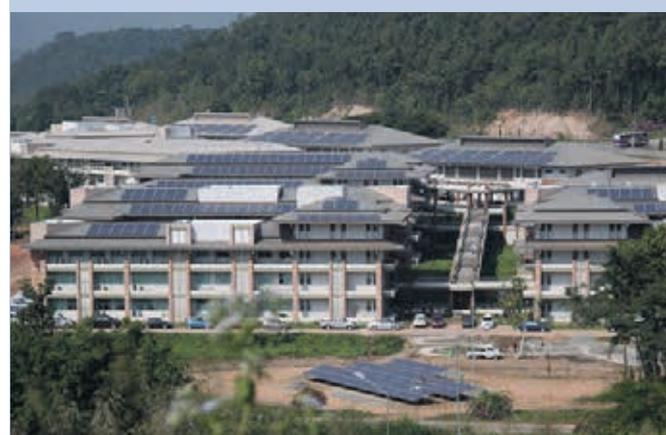
Fig. 2 - 500 kWp PV Rooftop of the Smart Grid System at the University of Phayao (Photos: University of Phayao).
