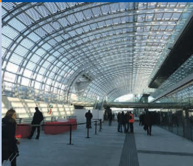
Fig. 2 - BIPV plant in Torino, 553 kWp, monocrystalline modules
