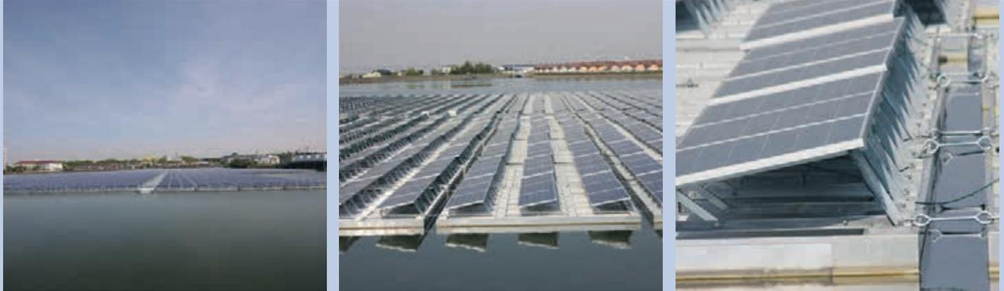
Fig. 1 - Floating PV Power Plant (INFINI Hyogo Daikyū Power Plant) (Inami Town, Hyogo Prefecture). Multicrystalline silicon PV module: 250 W x 6 846 modules (by INFINI) 1,7 MW.
