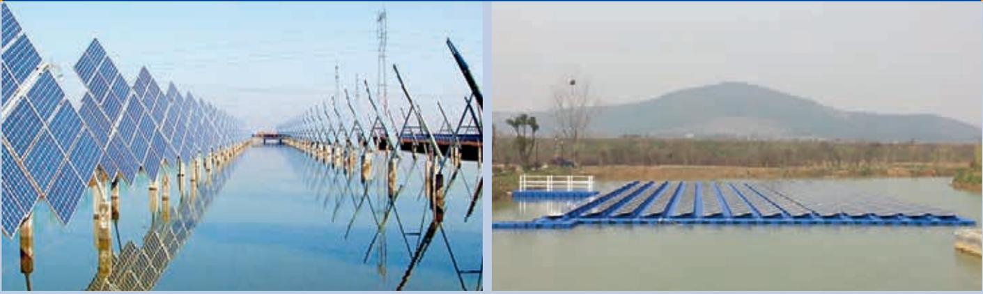
Fig. 2 - Fish-Pool PV and PV on Water Surface.
