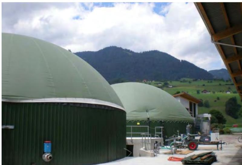
*Figure 13: Biogas plant in Kägiswil, producing annually 1.5 GWh electricity and 1.7 GWh heat.*
