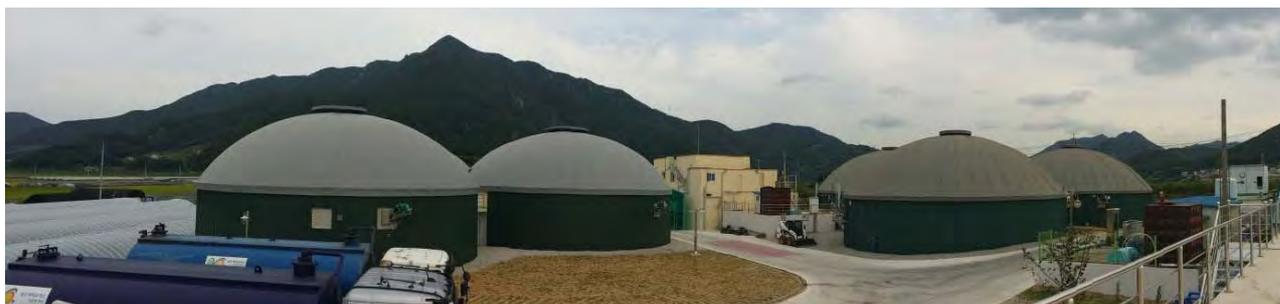
*Figure 11: Yangsan Biogas Power Plant that is producing 1.0 GWh electricity (with 2.3 million Nm<sup>3</sup> biogas) annually. (source : Kyungnam Province, Korea)*
