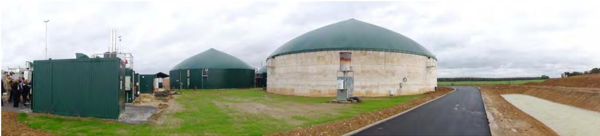
*Figure 6: Biogas unit in Chaumes en Brie, France, owned by Bioénergie de la Brie Co. The plant produces biomethane and various products from agro food biowastes and manures. The biomethane is injected into the natural gas grid and feeds 5 cities located close to the unit.*
