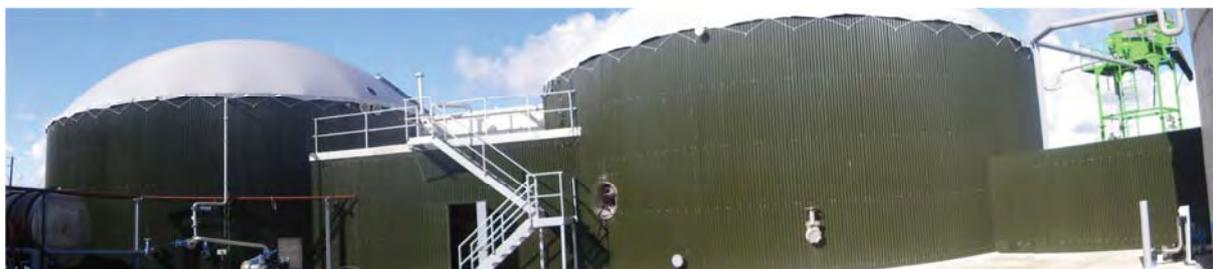
*Figure 10: Biogas plant McDonnell Farms Limited. Primary Digester and first covered storage digester. David McDonnell milks 300 dairy cows in Limerick and also operates a free range poultry farm. In 2009/2010 he installed the most modern farm digester in Ireland which has a capacity of 250 kWh<sub>e</sub>. (Source: SEAI (Sustainable Energy Authority of Ireland) Anaerobic Digestion: A case study – McDonnell Farms Biogas Limited, Shanagolden, Co. Limerick))*
