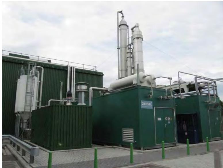
*Figure 15: The biogas plant owned by De Meerlanden Rijsenhout that is producing green gas, CO<sub>2</sub>, heat, compost and water*
