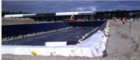
AGRU for many years has supplied PE pipes for hot water applications. With this vast knowledge and experience AGRU developed the first high temperature resistant (HTR) PE geomembrane in the marketplace. It looks, feels and welds like every other HD-PE geomembrane. Additionally it offers an outstanding
